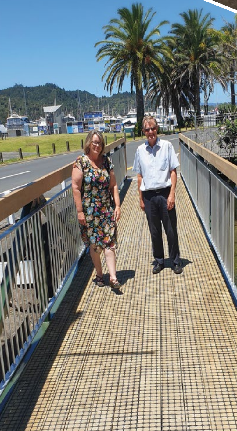
Waikino Gorge Hauraki District Council 12m pedestrian bridge
